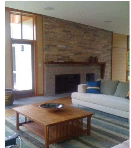
Glass doors on the fireplace reduce toxic air from filtering through the residence.
